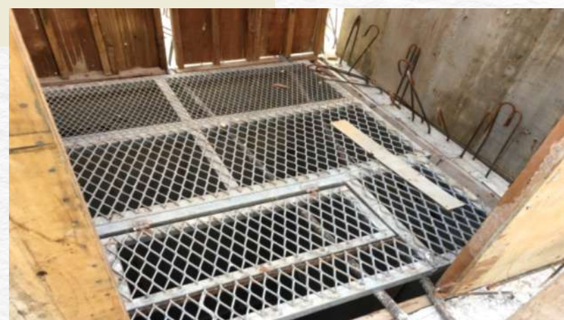
Elevator shaft steel construction platform
