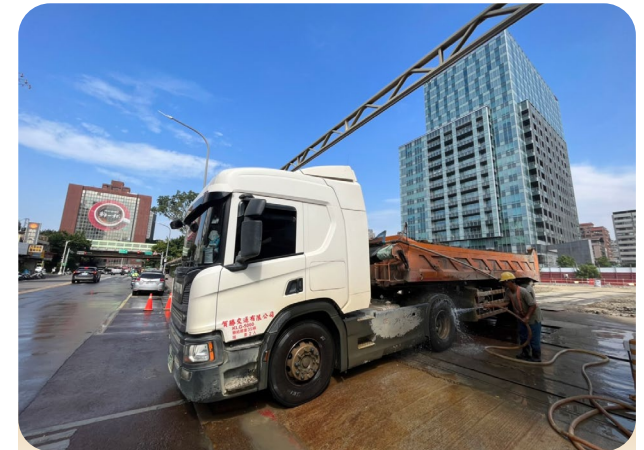
Vehicles are thoroughly washed before leaving the construction area
